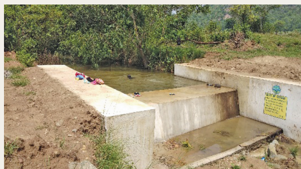
VSS members using the Check Dam-02
