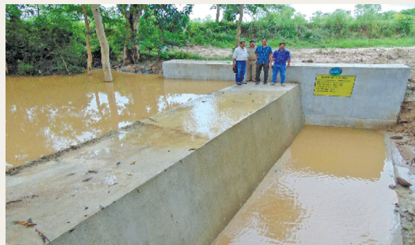
I/C RCCF-Cum-FD STR, Baripada & DFO-cum-DMU Chief, Baripada, visiting the Check Dam-01
