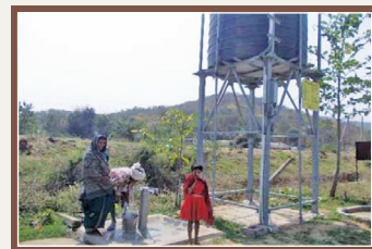
Drinking water facility at Balipata VSS
