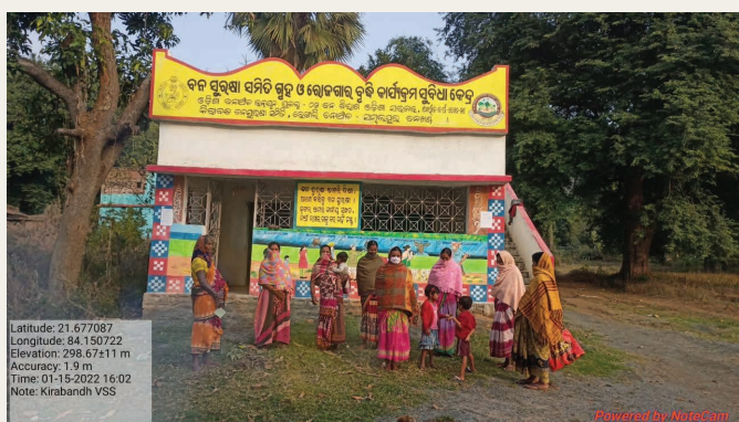
VSS building -cum-IGA Centre, Kirabandha VSS, Sambalpur DMU
