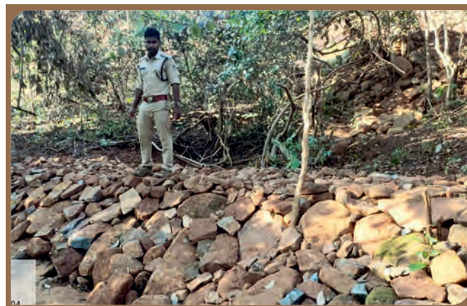
LBCD work at Raidiha VSS in Keonjhar Division
