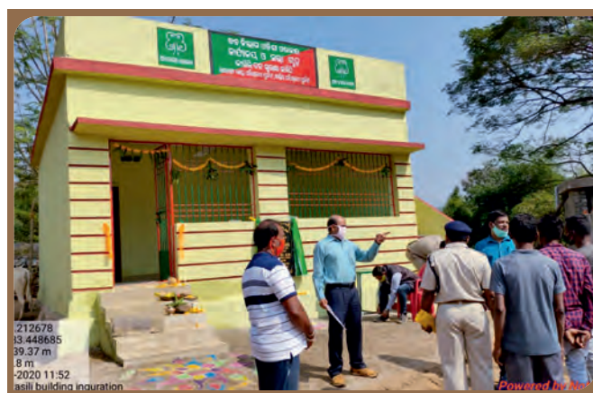
Kasili VSS Building, Rayagada Division
