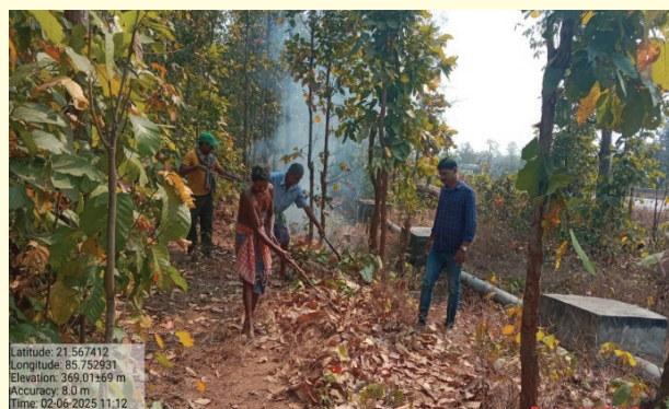
Fire Line creation work at Pipalia VSS, Keonjhar Division
