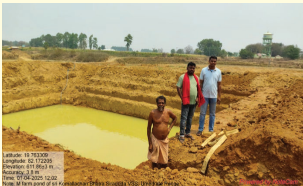
Farm pond support to VSS members through convergence at Siraguda VSS, Nabarangpur Division
