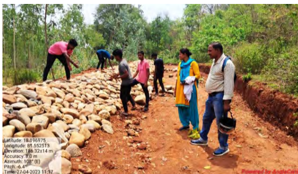
LBKD restoration Work At Tegadapalli Vss Kalimela Range of Malkanagiri Division
