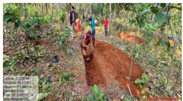
Restoration of Staggered Trench at Ranipada VSS, Keonjhar WL Division
