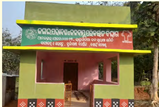
Bhalugadia VSS Building under Kuliposh FMU of Bonai Division
