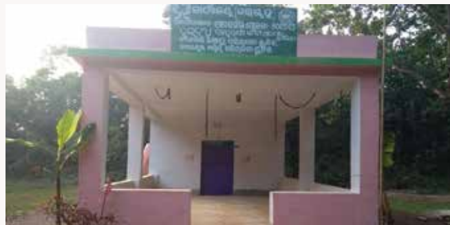
Duibandhu VSS building constructed under AJY Scheme
