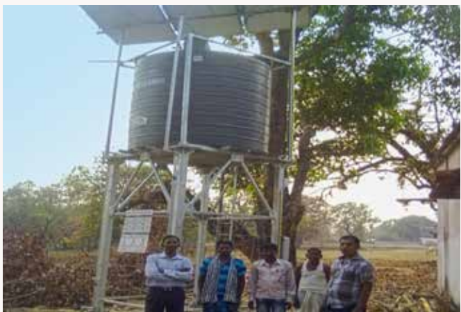
Solar Energy Based Drinking Water Supply at Arjunchuan VSS
