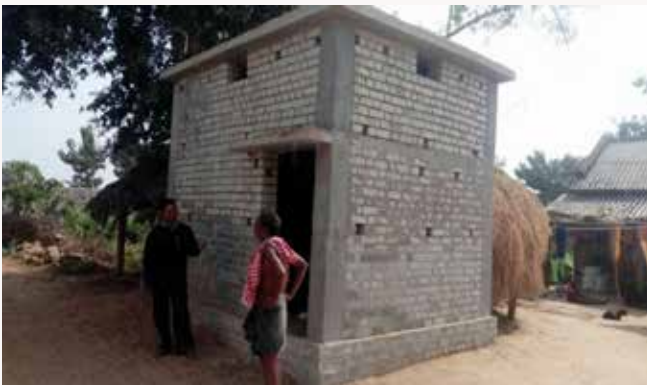
Construction of Maa Mangala Pitha in convergence with MLA LAD Fund
